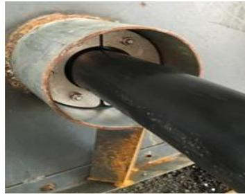
Figure 4. Use of seal for the cable entry hole
