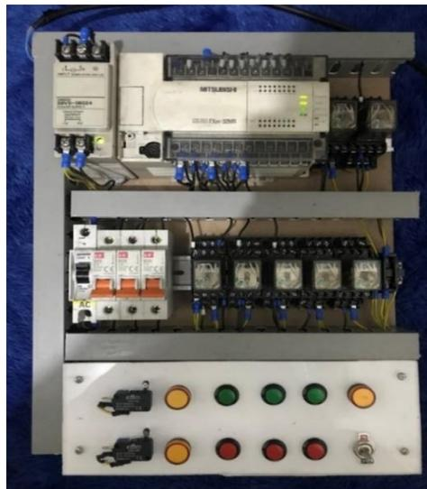
Fig. 8. PLC Control Panel
